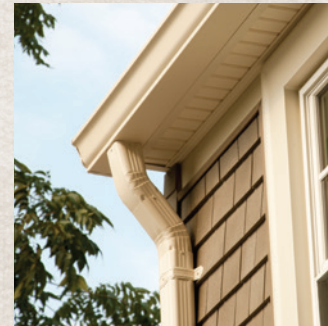
Rainware, Fascia, Soffit
