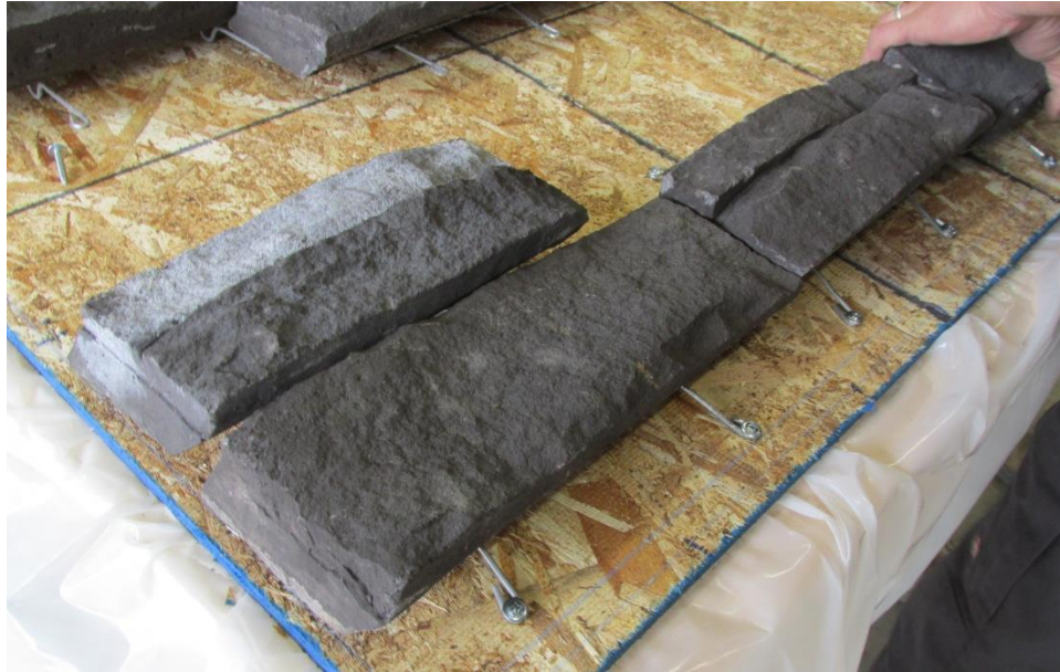
Figure 8: Attaching the First Row of ClipStone (Fastened both above and below the ClipStone)
