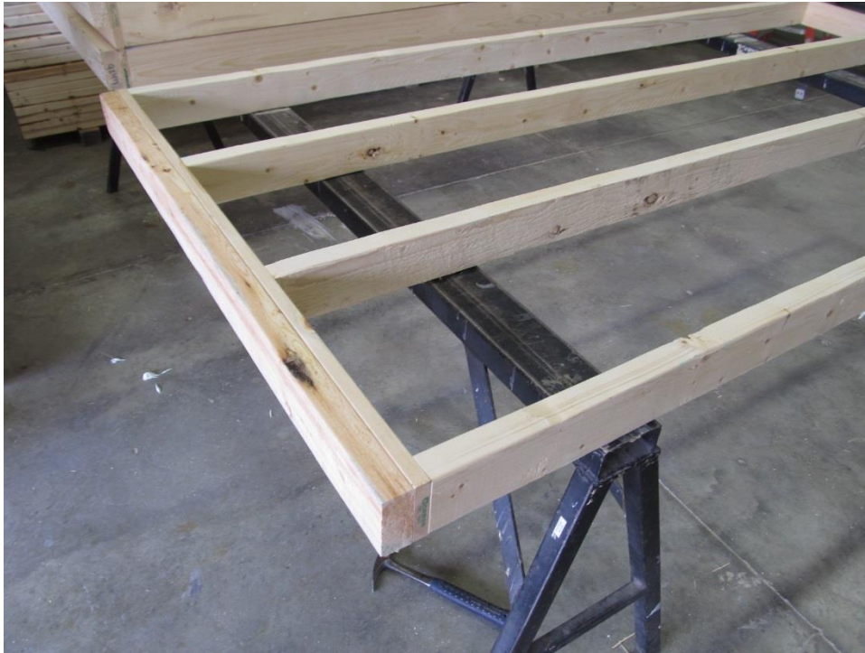
Figure 6: Construction of Wood Framing
