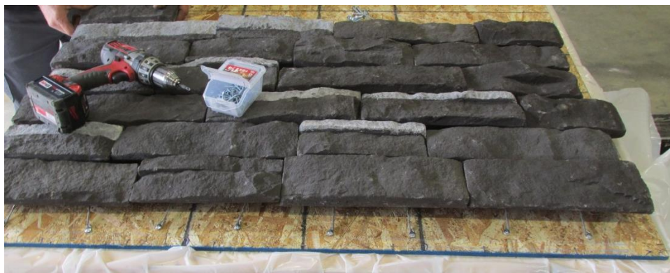
Figure 10: Continuing to Attach Rows of ClipStone (All rows above the first row were only fastened above the ClipStone)
