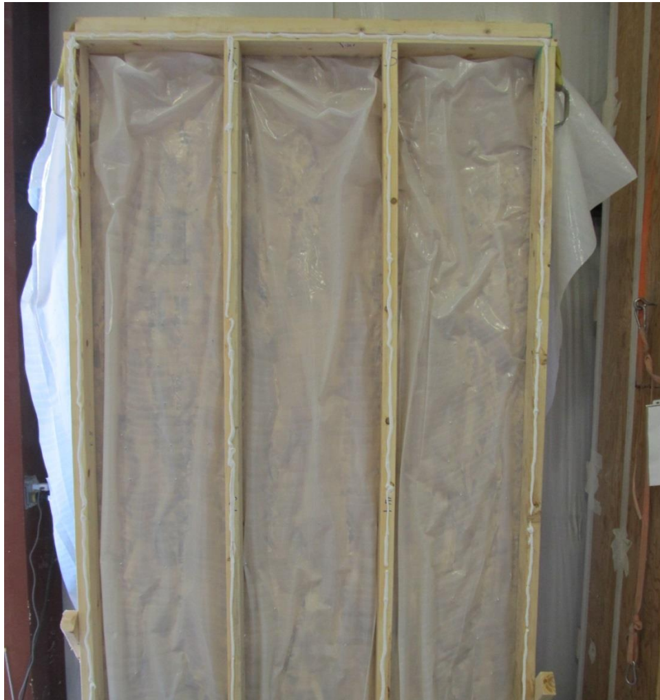
Figure 12: Adhesive Application to Interior of Wood Framing
