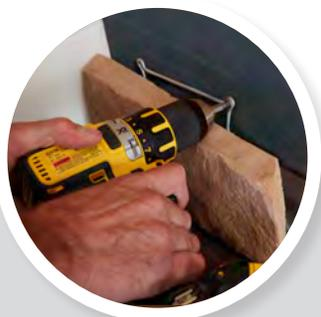
**1** Simply prep the wall, place a screw in each eyelet and attach ClipStone to the wall.
