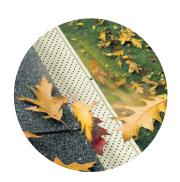
Leaf Relief products do not cause ice dams. If icicles form on roof edge, check the attic for proper ventilation and thermal insulation.
