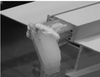
5. Align head jamb to side jamb, and push them together until the frame corner key is properly seated into both the head and side jamb cladding. Fasten the frame cladding with (2)  $\#6 \times 1-1/2$ " flat head screws. Seat screws evenly on opposite sides to ensure proper alignment of the corner joint – this is critical to the performance and appearance of the finished door unit.
