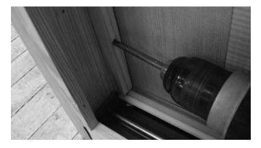
19. Install the head inactive panel stop, and fasten in place with #6  $\times$  1-1/2" flat head screws. The stop should be justified to the side stop previously installed, and should fit all the way down square in the groove in the side jamb.
