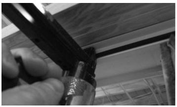
23. Install the 3/4" x 1-1/2" x 1/4" black foam blocks to the top and bottom ends of the interlock as shown. The adhesive side of the block should face the head or sill, not the interlock.
