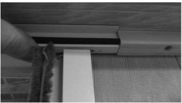
22. Fasten the vinyl parting bead in place with 1/2" x 1/2" staples as shown. Place one staple about 2"- 4" from each end, and 8"- 10" on center in between. (Small flat-head screws may be substituted for the staples, as long as they don't interfere with operation of the active panels. You can also use caulk/sealant as an adhesive.)
