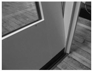
15. Stand the panel up. Bow the head jamb up slightly (if necessary) to clear the top of the panel.
