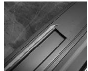
14. Using the correct panel for this side, and from the interior of the door opening - tilt the top of the panel towards you and set it onto the sill. Ensure that the sill locator on the bottom of the panel fits into the groove on the sill. The side of the panel should be all the way against the side jamb.
