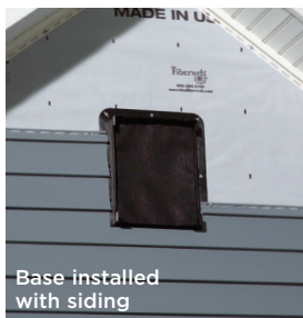
Vent Cap installed after siding is finished
