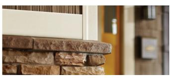
Tapered Sill Window sills and transition between siding materials
