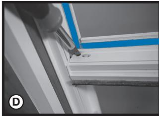
**STEP 3.** Reinstalling the meeting rail. Align the meeting rail with both jambs and slide the meeting rail over the bottom anchor tabs then rotate the rail over the top anchor tabs to fully engage the anchors **(Figure E)**. Place original screws back in their original holes and tighten – DO NOT OVER TIGHTEN.
