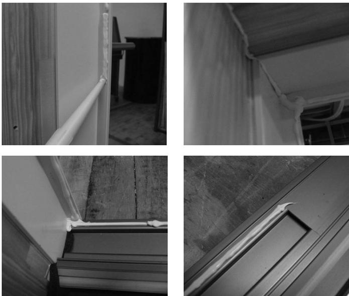
14. Using the correct panel for this side, and from the interior of the door opening - tilt the top of the panel towards you and set it onto the sill. Ensure that the sill locator on the bottom of the panel fits into the groove on the sill. The side of the panel should be all the way against the side jamb.
