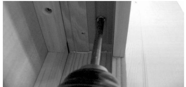
30. Install the panel bumpers to the unit by clipping the rubber profile over the rail in the sill (an alternate at the preference of the installer is to apply them to the head of the unit, fastened in place with a screw.)
