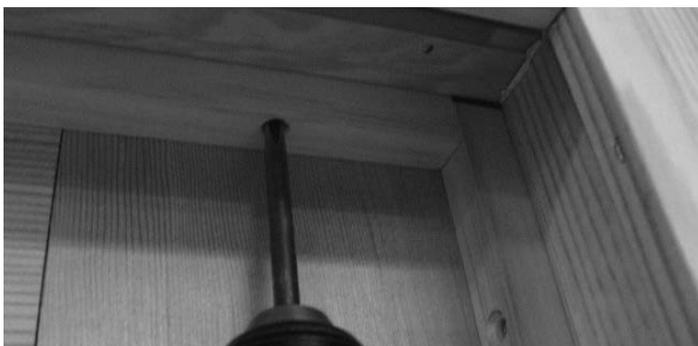
23. Install the 3/4" x 1-1/2" x 1/4" black foam blocks to the top and bottom ends of the interlock as shown. The adhesive side of the block should face the head or sill, not the interlock.
