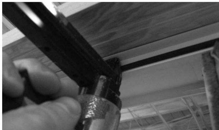
19. Install the head inactive panel stop, and fasten in place with #6 x 1-1/2" flat head screws. The stop should be justified to the side stop previously installed, and should fit all the way down square in the groove in the side jamb.
