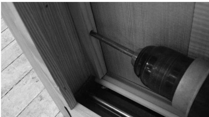
22. Fasten the vinyl parting bead in place with 1/2" x 1/2" staples as shown. Place one staple about 2"- 4" from each end, and 8"- 10" on center in between. (Small flat-head screws may be substituted for the staples, as long as they don't interfere with operation of the active panels. You can also use caulk/sealant as an adhesive.)
