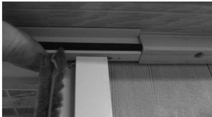
18. Install the side inactive panel stop, and fasten in place with #6 x 1-1/2" flat head screws. The stop should be justified to the top of the jamb, and should fit all the way down square in the groove in the side jamb. (It may be easier to start at the bottom of the side jamb and work your way up.)
