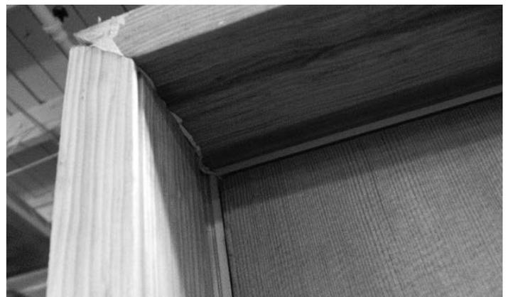
17. Fasten the panel in place through the holes use the bracket at the top of the panel. Use #6 x 3/4" stainless steel screws.
