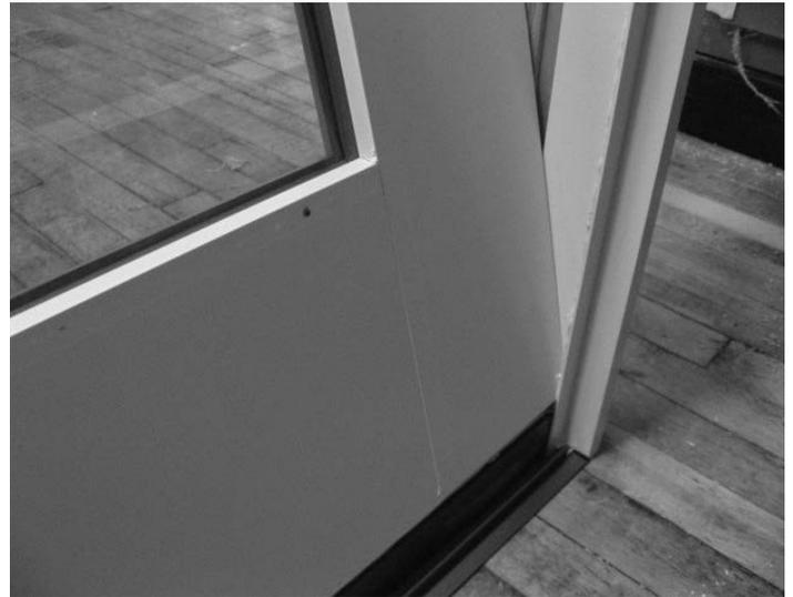
15. Stand the panel up. Bow the head jamb up slightly (if necessary) to clear the top of the panel.
