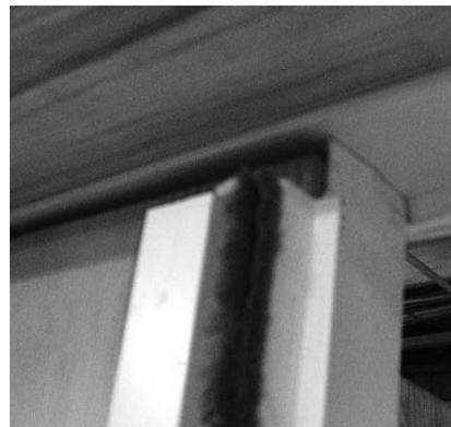
16. On the exterior, check again to make sure that the panel is properly seated in the sill, so that no space shows between the bottom of the panel and the sill. From the interior, check to make sure that the panel is seated evenly against the side jamb.
