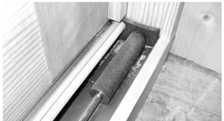
31. Install the self-adhesive, foam wedge pad in place at the bottom of the astragal as shown.
