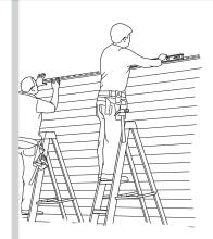
Fasten a maximum of 16" on center; fastened straight and level to prevent distortion of the panel. Start nailing in the middle of the panel.
