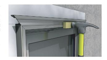
**1g) (Required)** Fasten each top corner by driving a #6 x 1½" Flat-head screw through the predrilled hole in the head casing into the screw boss in each side casing. Be careful to maintain proper alignment of parts when starting and tightening the screws.
